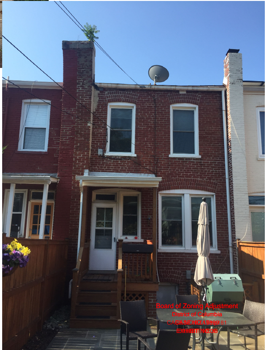
EXISTING REAR FACADE
